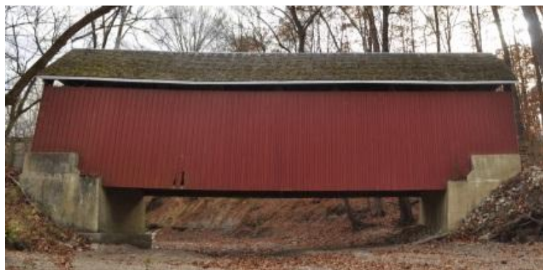
Figure 3.2: Different views of the Zacke Cox Bridge
