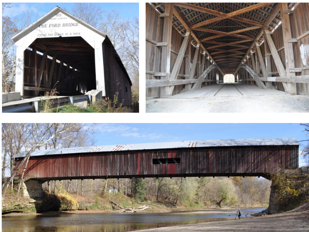
Figure 3.18: Different views of the Cox Ford Bridge
