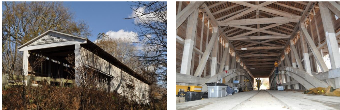
Figure 3.9: Different views of the Portland Mills Bridge
