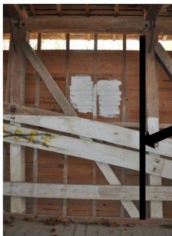
a. Vertical skew of the vertical members
