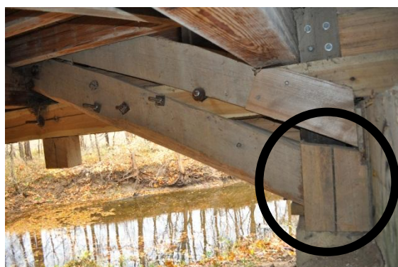
b. Alterations to the arch and abutment interaction
