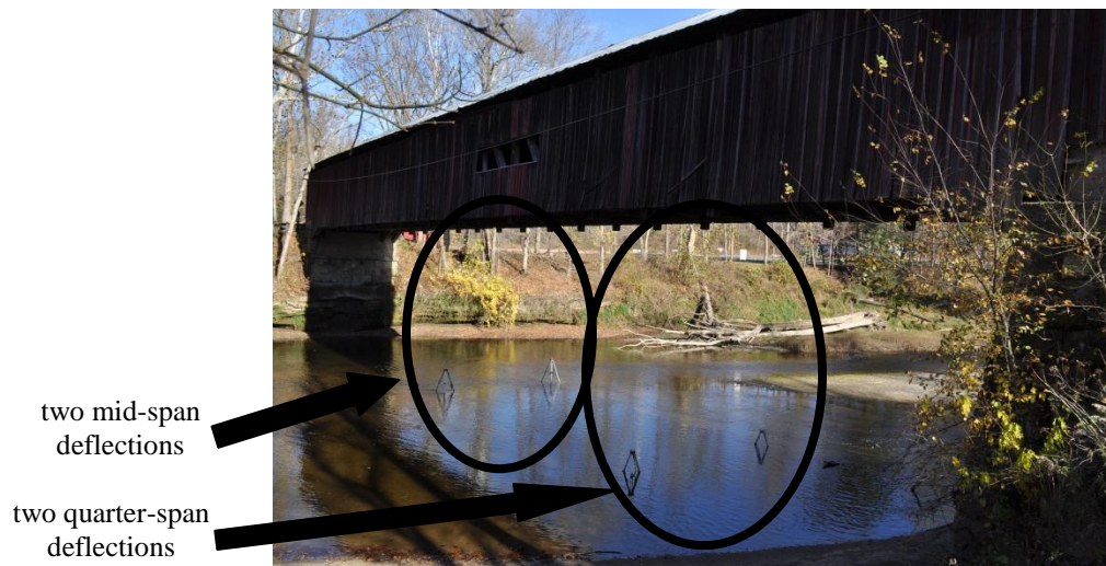
a. Displacement gauges and tripods for mid-span and quarter-span deflection measurements on both trusses
