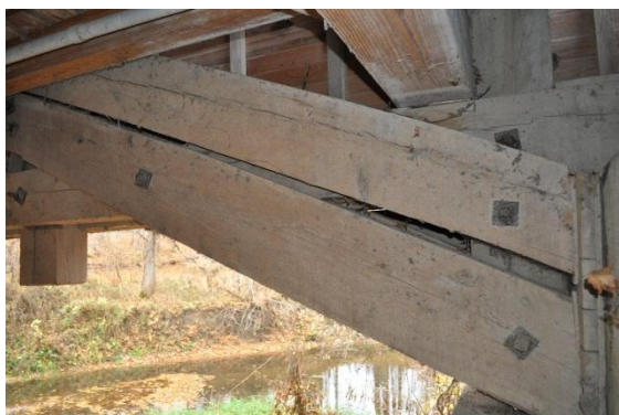
b. Alterations to the arch and abutment interaction
